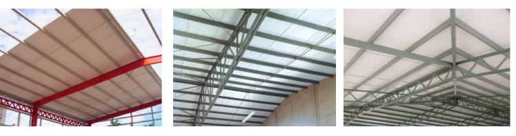
BPA INSULATION (REINFORCED ALUMINIM + 3/16" POLIETHYLENE BUBBLE + REINFORCED ALUMINIUM) DIMENSIONS AND TOLERANCES OF THE STANDARD PRODUCT
